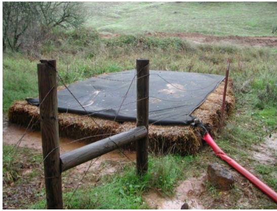
Figure 3.HYDRO.a-01: Typical Setup of Sediment Capture Bag
